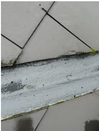
valley coated in fibre paint.
