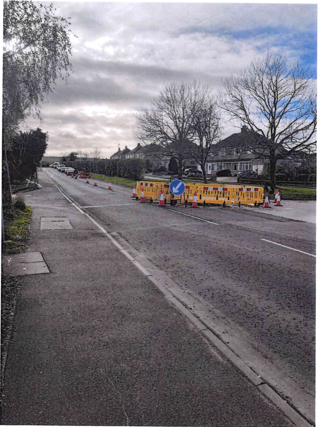
PHOTO2 : Showing the A4361 Swindon Road south bound. The operator entrance is to the left opposite the temporary road works.
