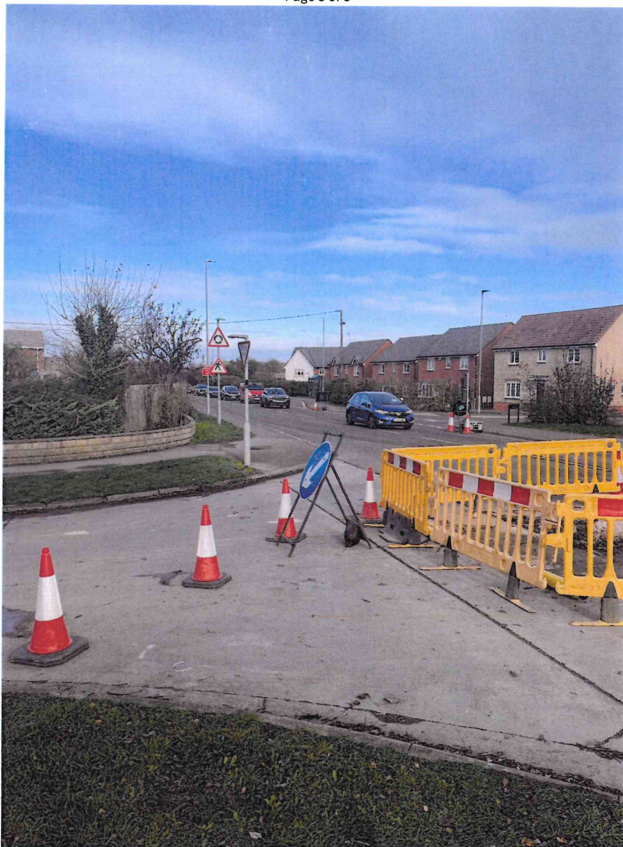
Photo 5: Taken opposite the operator site entrance looking north up the A4361 Swinson Road. The roadworks seen were very much temporary and were planned to be there for 1 day only .
